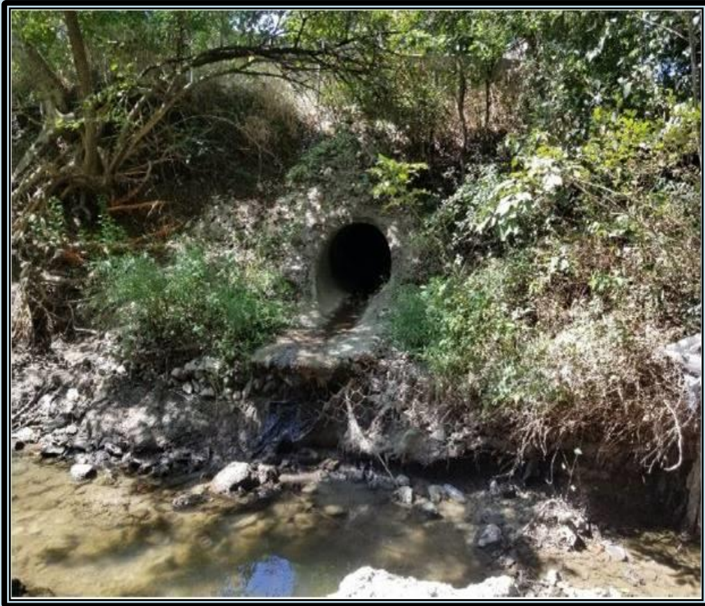
4105 Scott Drive Site
